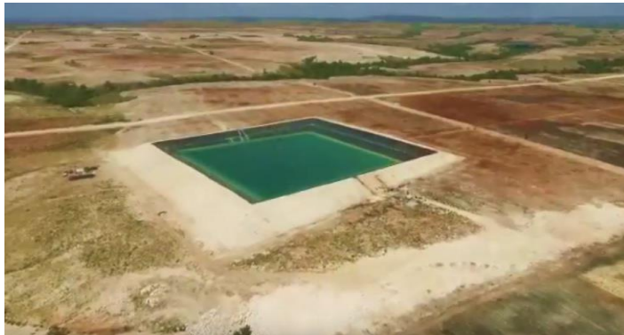
3. After water reservoir construction
