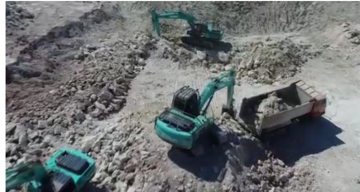
2. During water reservoir construction
